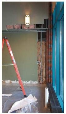
I worked with the electrician to add circuits so Campbell Inc. could install vent fans to draw warm air into the ceiling cavity to help prevent water in the pipes from freezing in the future.
