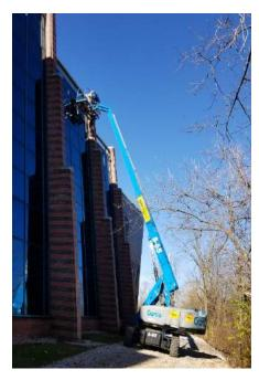
O'Neal Construction has finished the bottom sill of the window project. Here's a picture of them on the lift working on fascia near the roof, which is suspected to be a major issue with water leaking into the building.
