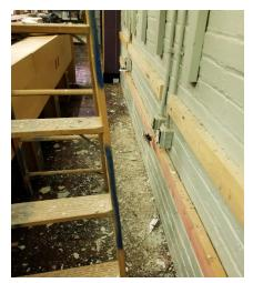
Terracon Inc. did some testing at Michigan Ave to look for the cause, and possible solution to the water entering the building through the basement walls. We had to remove shelving in preparation for the testing. Terracon recommended that we remove all loose paint on the north wall. After clean up we will get shelving back in place.
