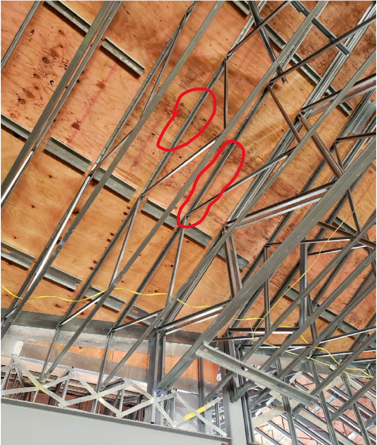
Examples of areas on the top chords where the fasteners don't appear to meet the required spacing.
