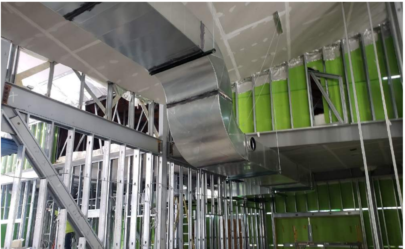
Main duct run above the staff area.
