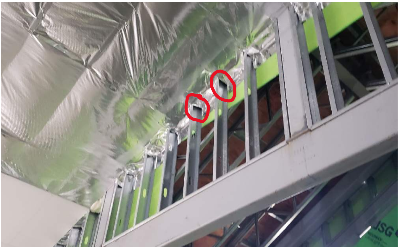
Foil needs to seal the inside of stud cavities and other gaps.
