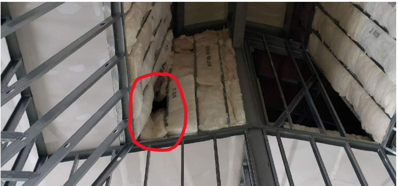
Batt insulation needs to stay in the stud cavity when drywall is installed.
