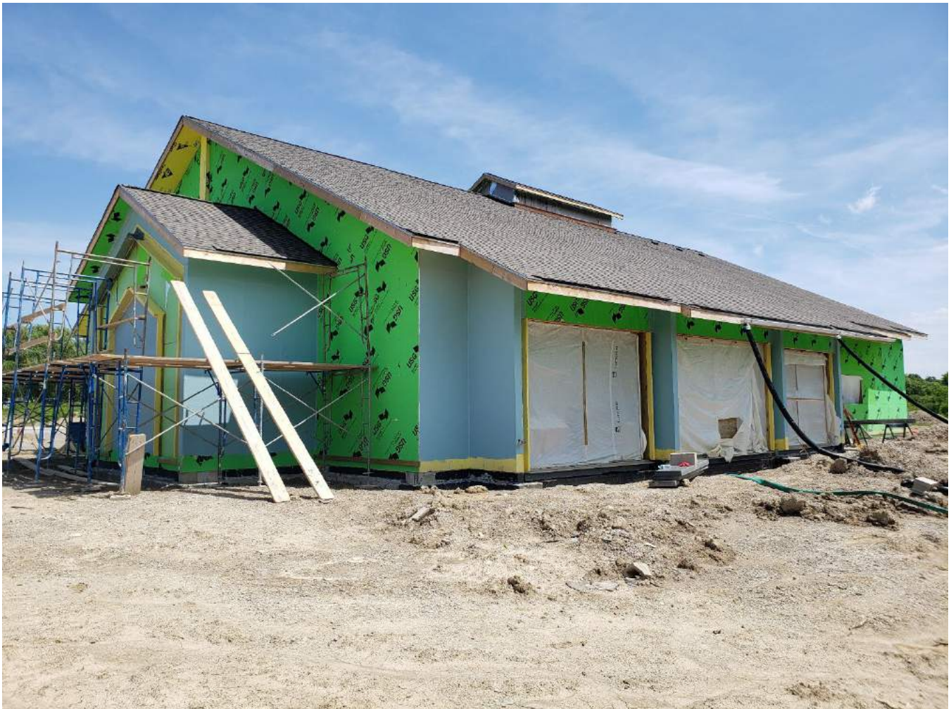
AVB (light blue) application has started on the exterior.
