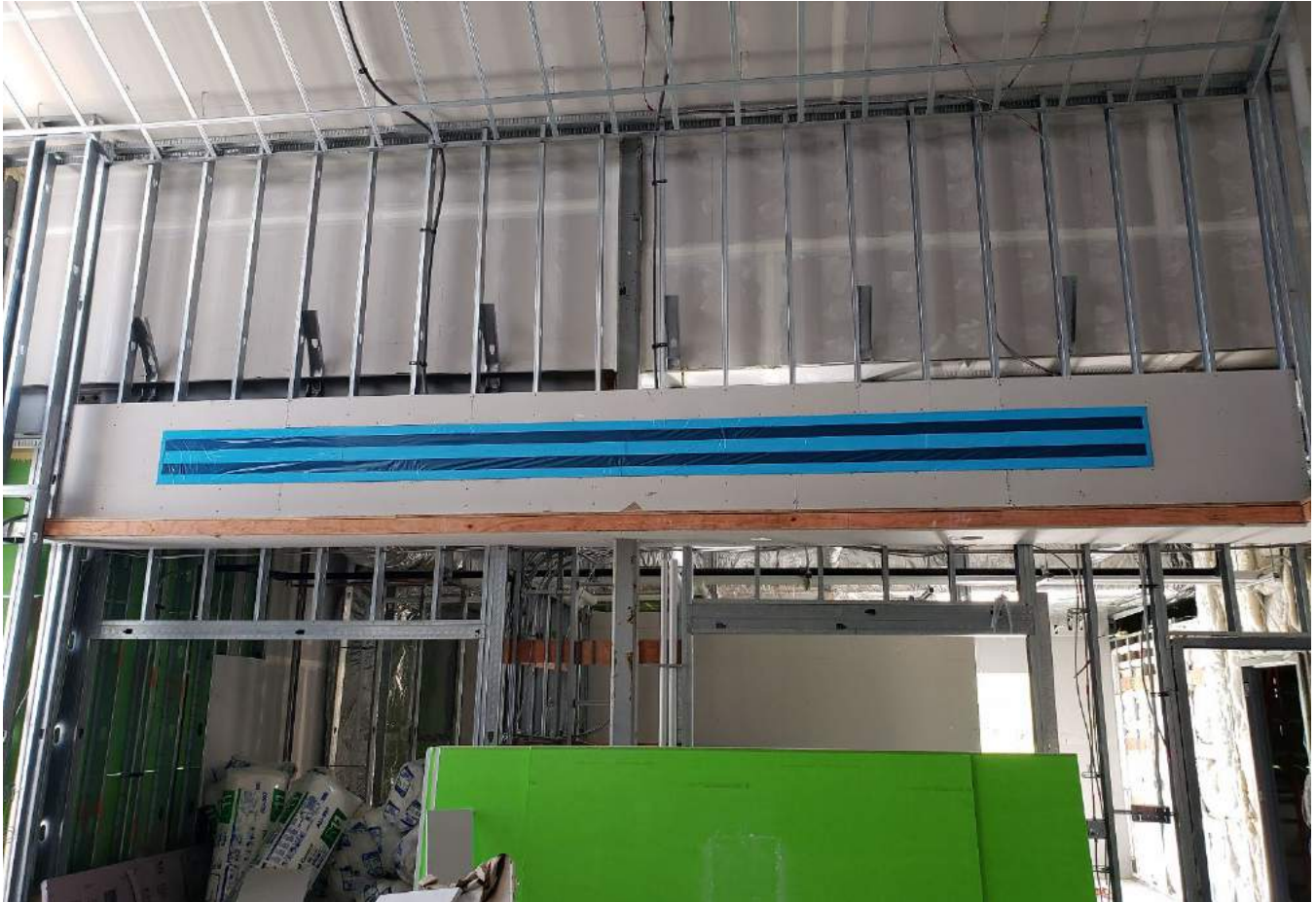
Horizontal grille opening in meeting room does not appear to match what is on the drawings, but it is centered at the correct height of 10'-10" A.F.F.
