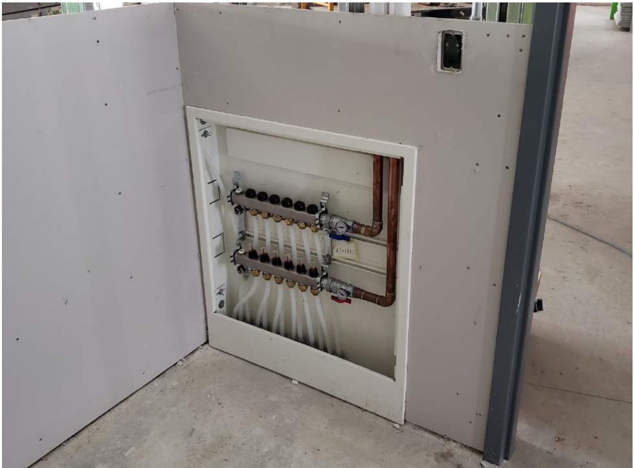
Radiant heating manifold installed in the corner of the staff area corridor; intent was that it would be closer to the door so that it isn't blocked by the shelving that will be installed in this area.
