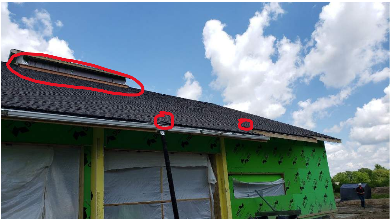
Gaps where shingles overlap eave vents, missing roof to wall vents at cupola
