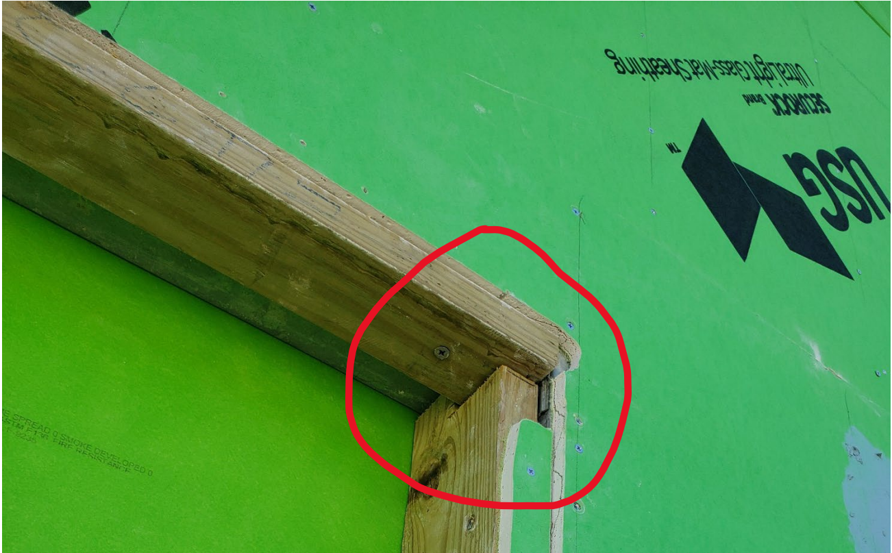
Header/Jamb framing.
