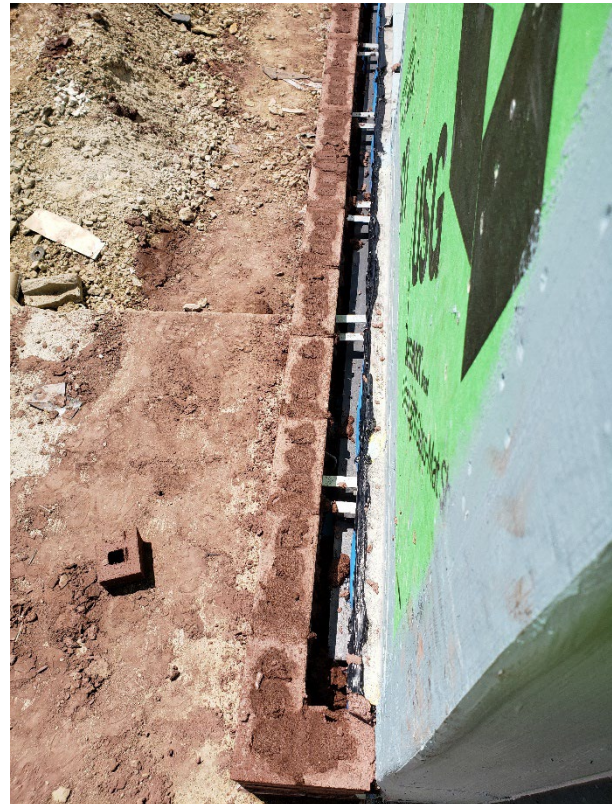
Insulation not installed tight to underside of masonry ties
