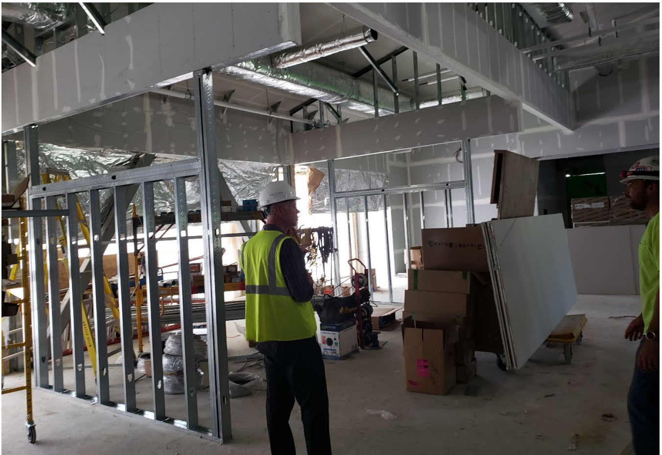
Framing at Teen Area wing walls.
