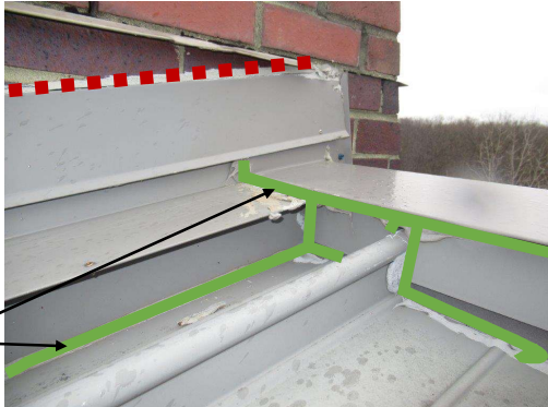
Photo 5- Typical Fin Scope
