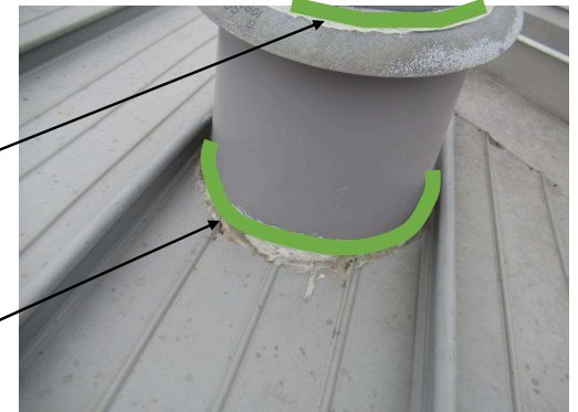
Photo 5- Typical Large Penetration
