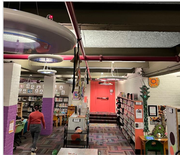
(R) Existing Fixtures which provide little downlight
