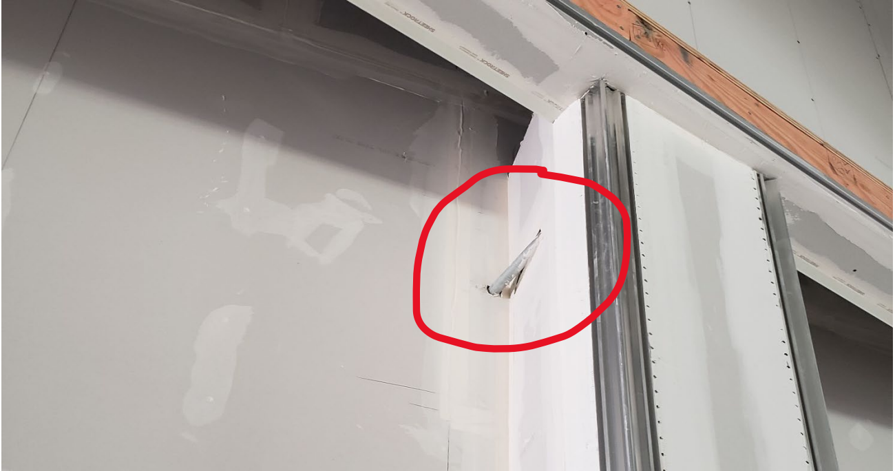
Exposed conduit at column B4
