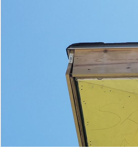
Warped nailers at the roof fascia.
