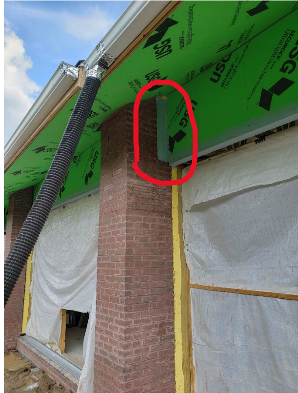
Gap in brick due to positioning of truss chord behind sheathing.
