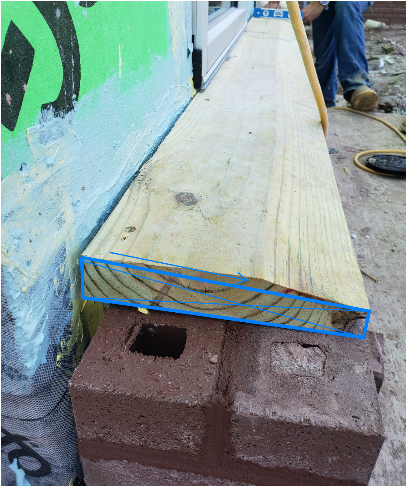
Blocking should be sloped over the whole width as shown in Arch details.
