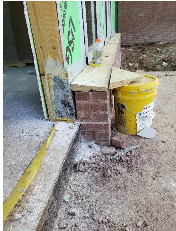
Corrected blocking with continuous single slope
