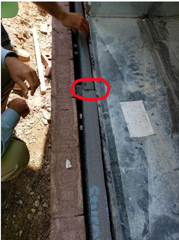
Spray foam to be installed at insulation gaps
