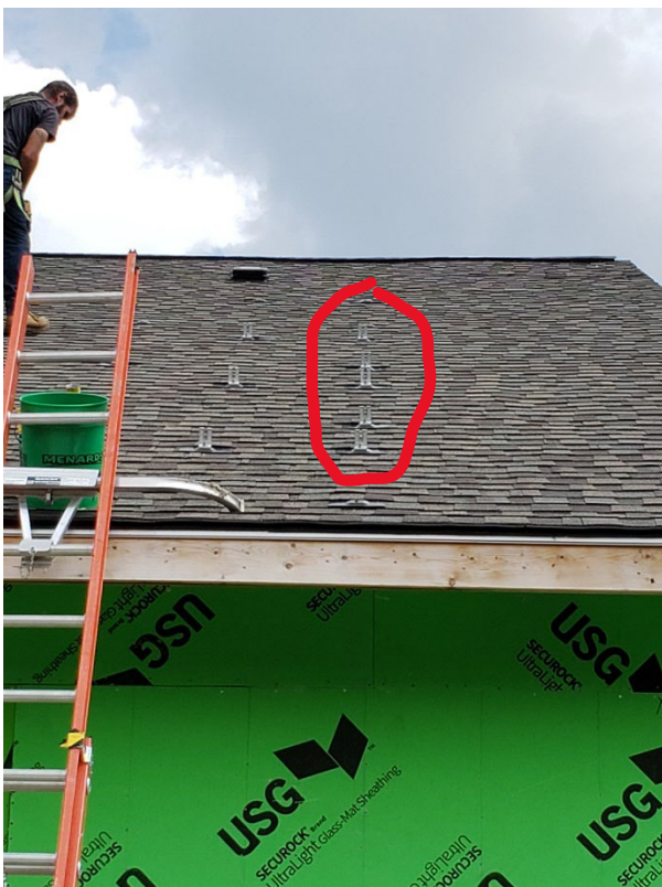
Solar bracket mounts not installed in a straight line
