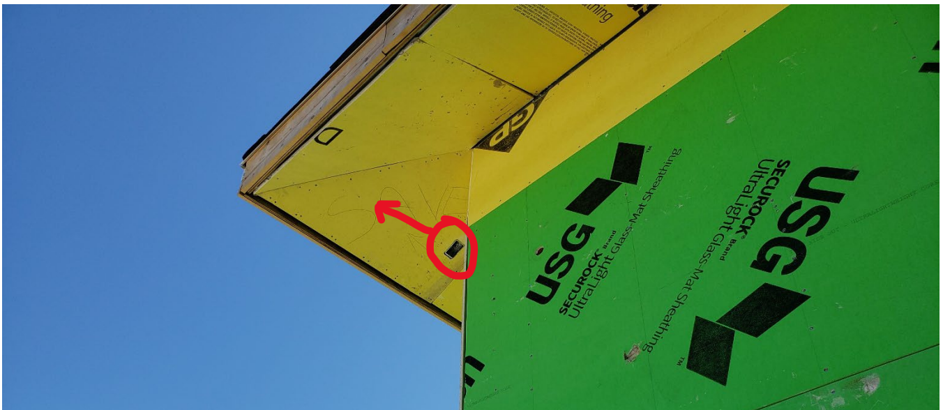
J. Box for camera may need to be moved for camera view angle.
