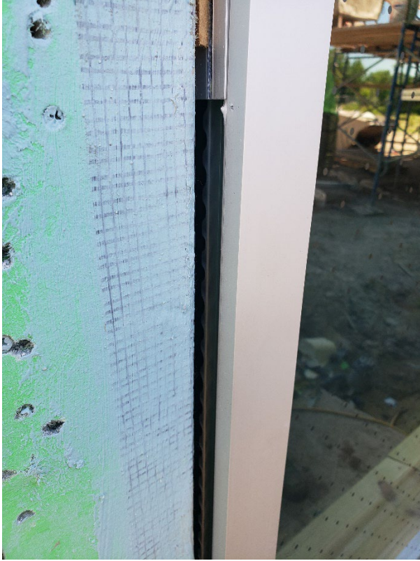
Gap at exterior windows, coordination needed
