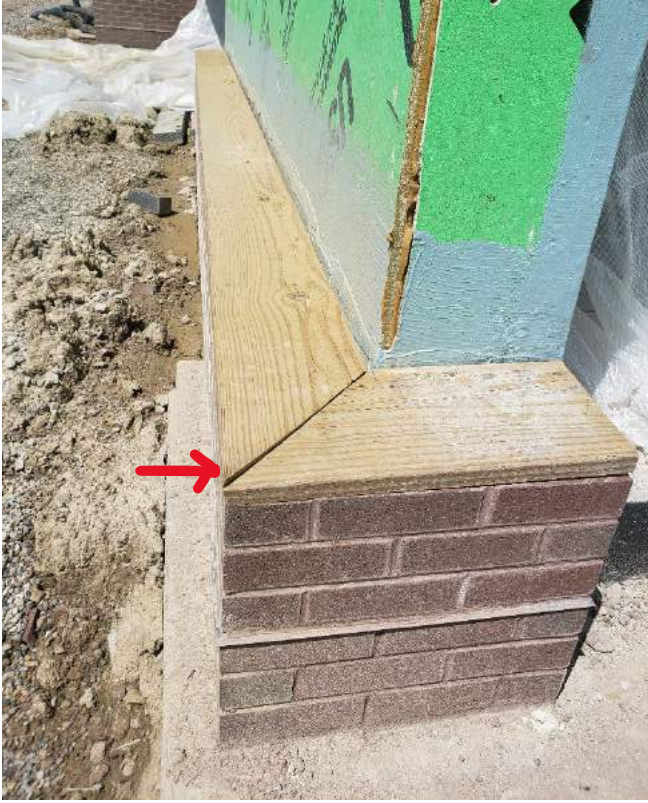
Warped blocking
