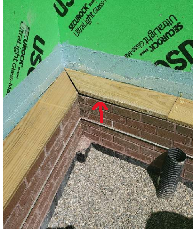
Warped Blocking
