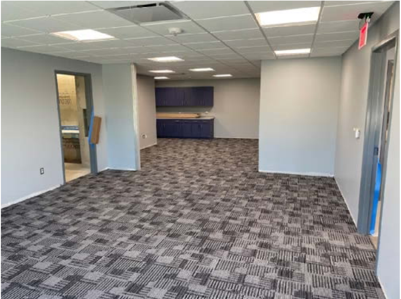
Carpet tile installed in the Staff Area.
