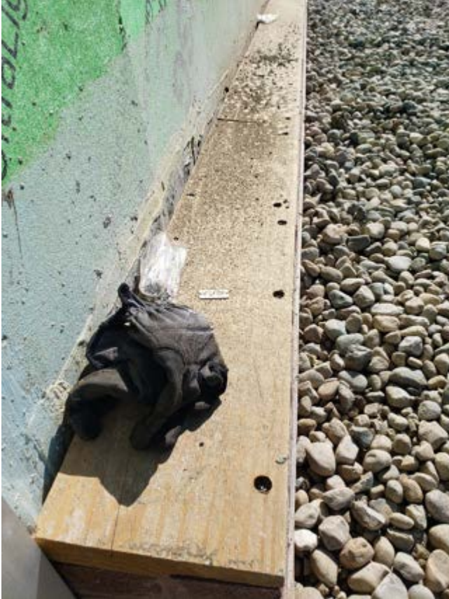
Blocking anchored into brick below
