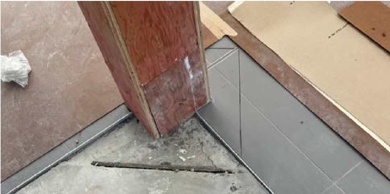
Cut Tiles at column CC2
