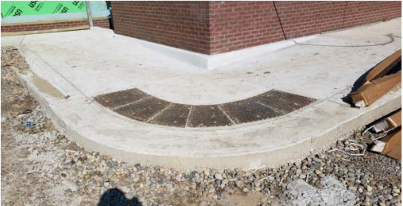
Cast iron tactile warning strip near mechanical screen wall.
