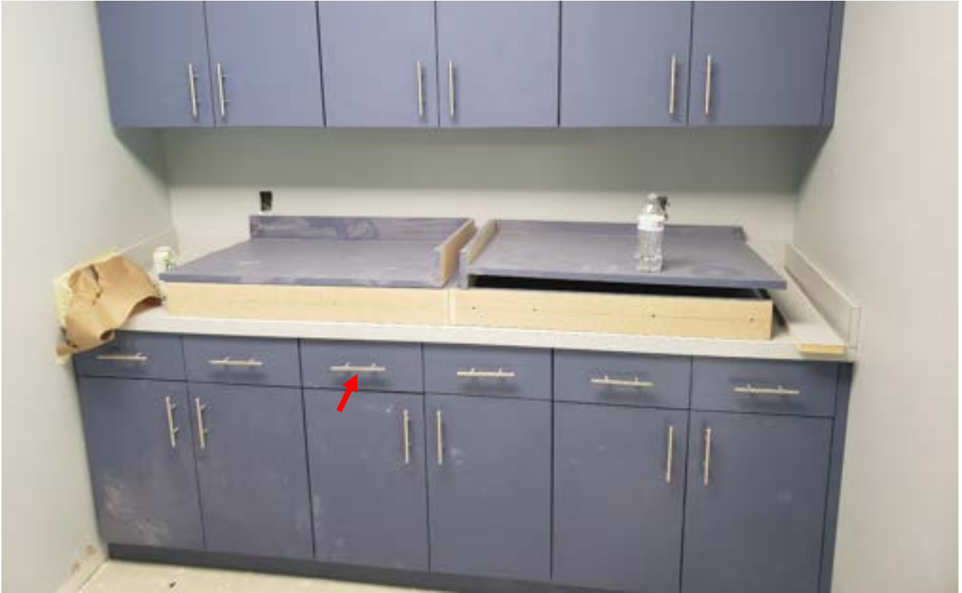
Cabinet doors have not been adjusted yet. Some of the hardware looks crooked and may need to be adjusted.
