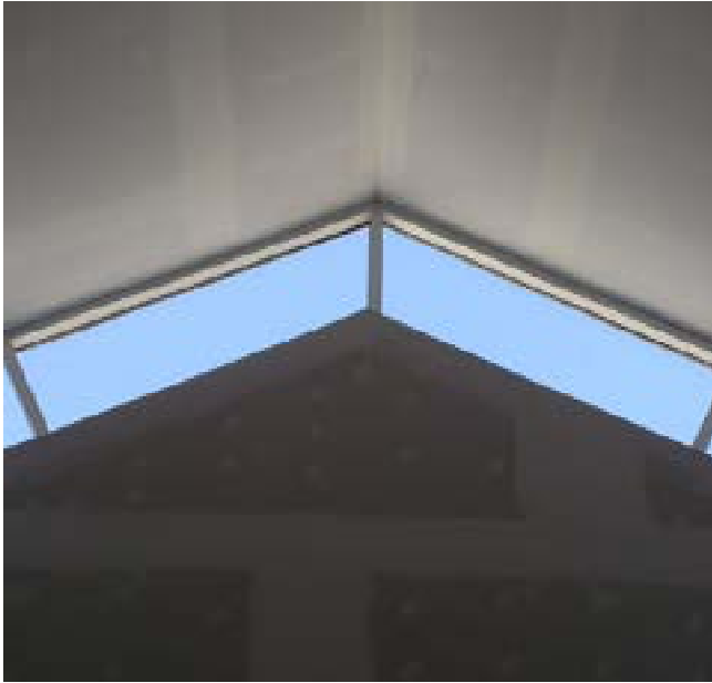
Off center drywall peak below glazing
