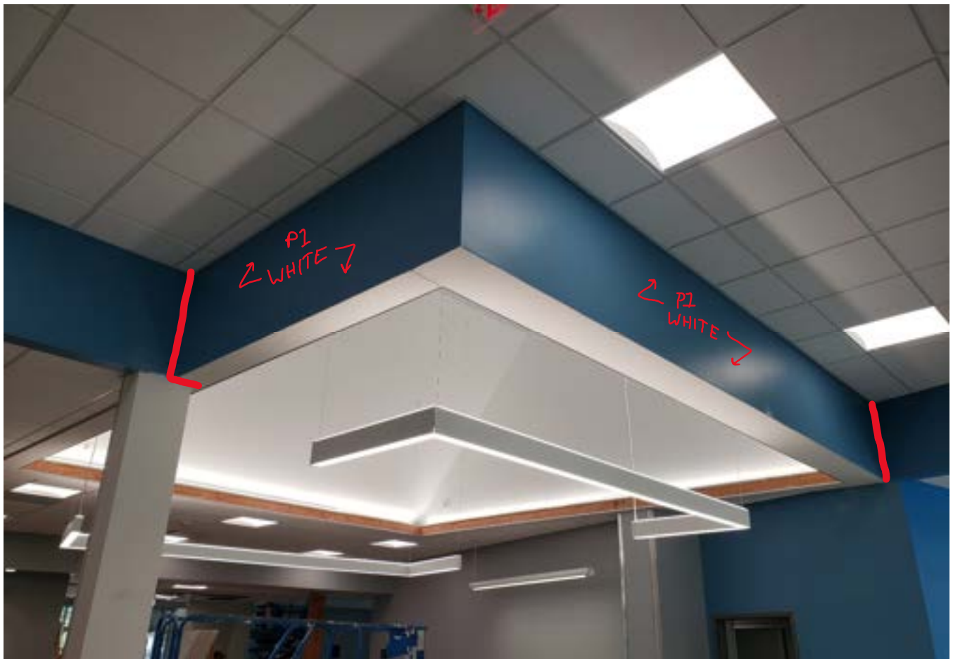
Soffit above the reference desk to be painted white as shown.
