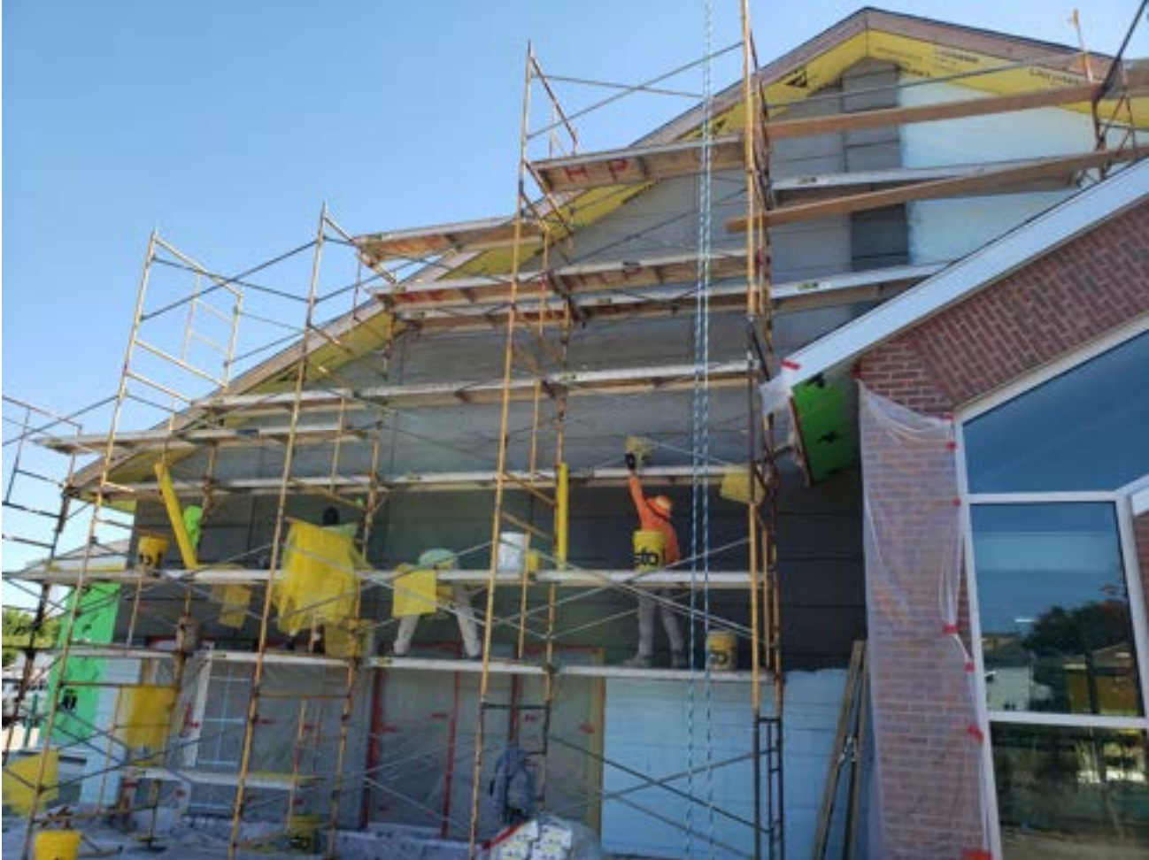
EIFS finishing on north face of the building
