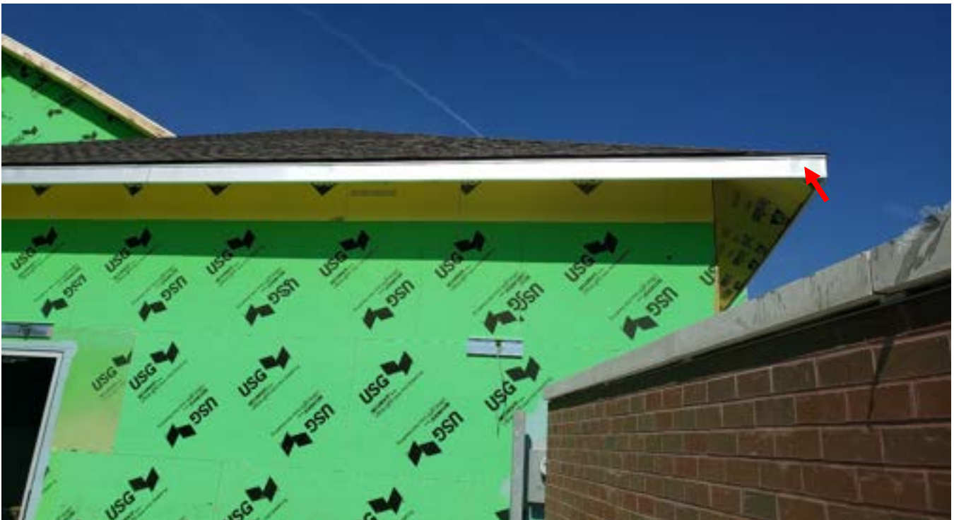
Metal fascia has been installed with exposed nails, causing some dimpling oil canning
