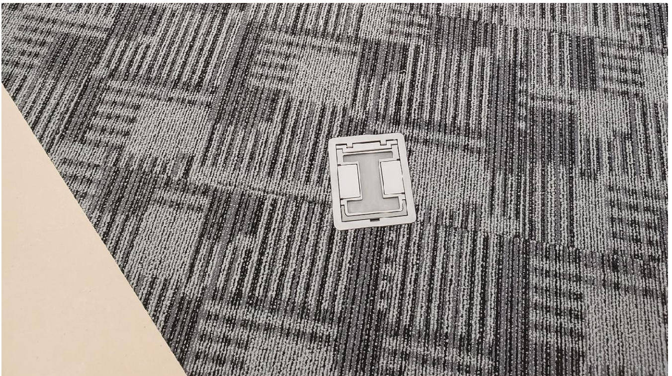
Carpet inserts in floor boxes to align with carpet tile orientation.
