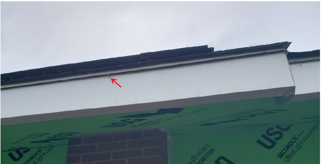
Loose nail at metal roof fascia
