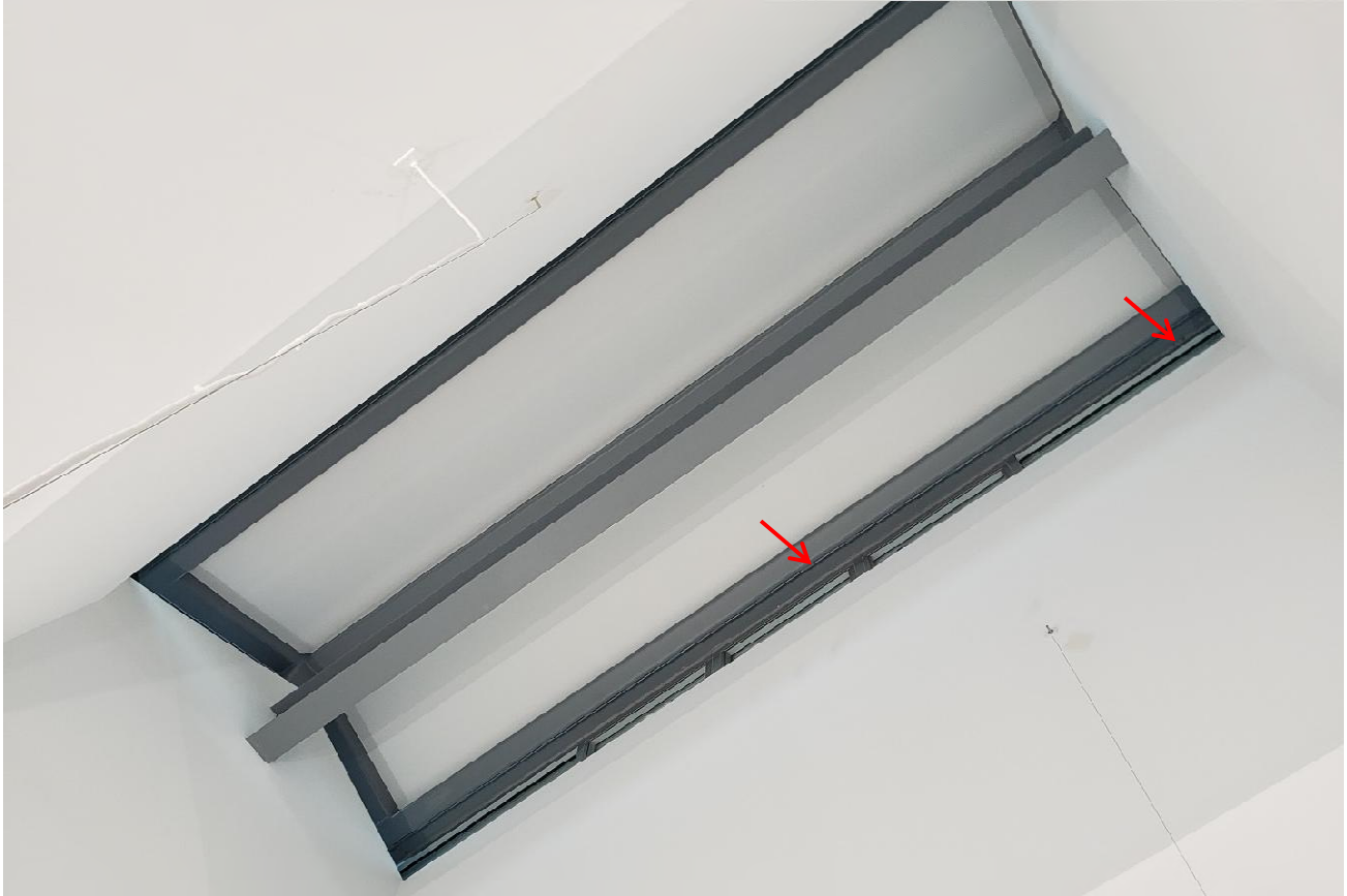
Touchups needed at cupola steel headers.
