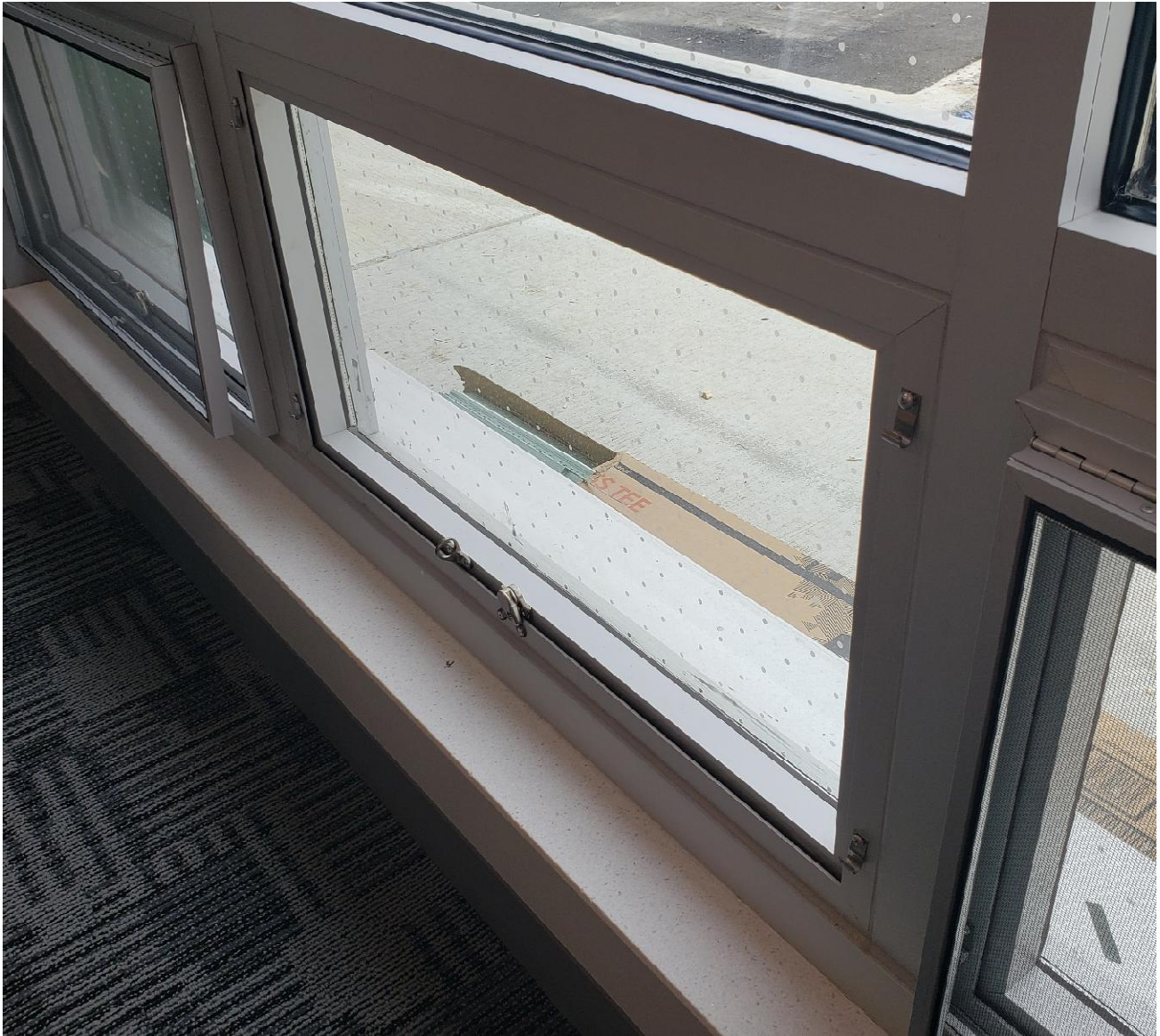
Clips for attaching screens at operable windows.
