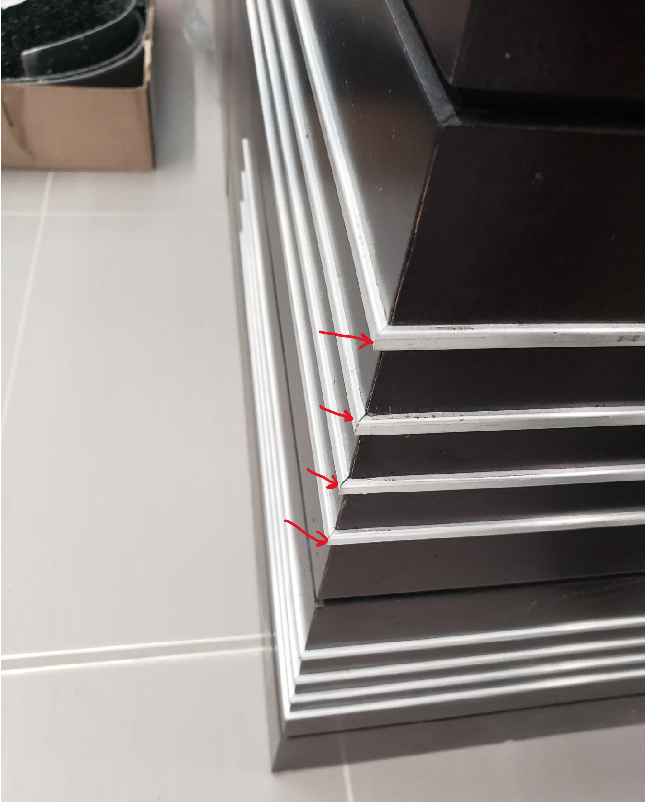
Edges of metal trim need to be eased, typ.
