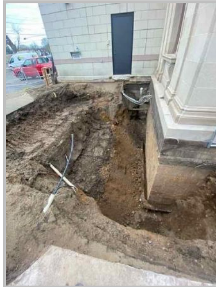
Left: Water sealing work in Spring '22 showing damaged conduit | Right: Location which power disruption was traced to by electrician Fall '22
