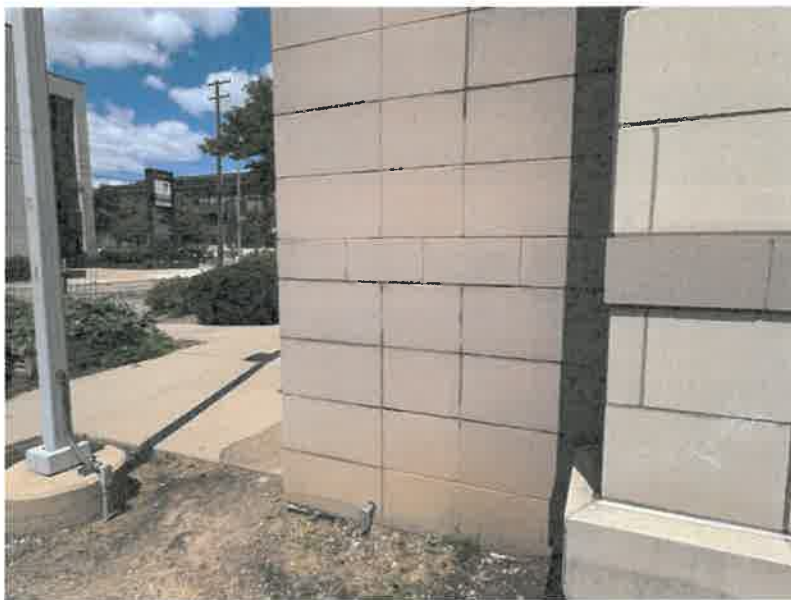
Varying dimensions of masonry units visible here will be replicated.
