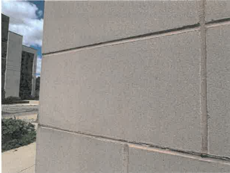
Closeup of cast rock units.
